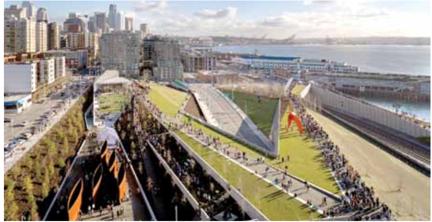
The Olympic Sculpture Park inserts a stable landform over remediated brown-fields, and zigzags to restore shoreline on the Puget Sound.
