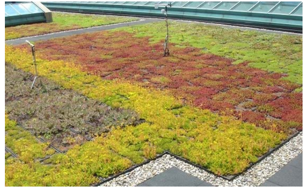
Figure 1: Photograph of the green roof modular system after one year showing above-grade monitoring stands
