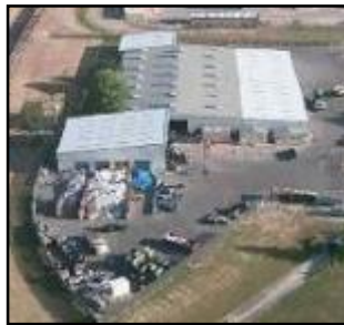
Fort Hood recycling center
