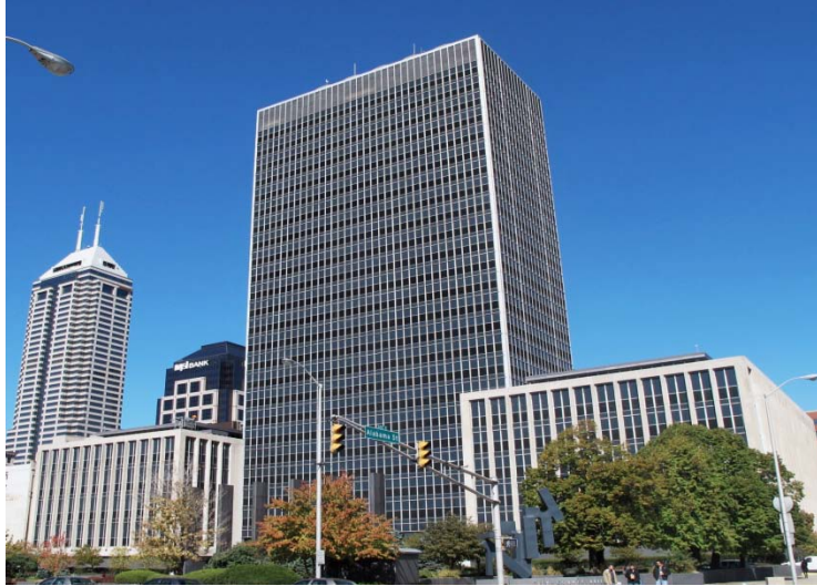
Indianapolis City-County Building (1962) 731,000 SF high rise ENERGY STAR rating 50 → 95 Cost: $11/SF
