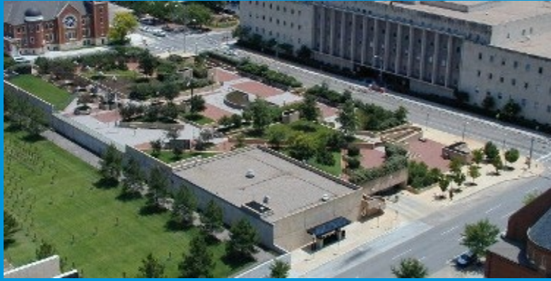
OKC Federal Parking Garage
