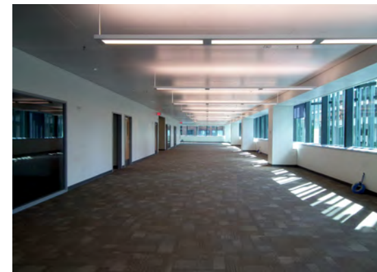
Image: Radiant ceiling panels
